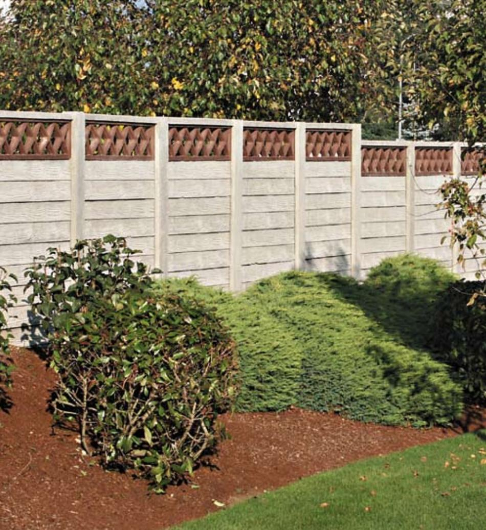
The fences simple design provides easy installation for contractors, landscapers and fence installers. The concrete posts are set into 12-inch diameter holes set five feet apart, posts are then anchored in a concrete footing. A bottom panel is then inserted down the post track and is supported by the concrete footing. Additional panels are stacked in one foot increments in an interlocking design.
